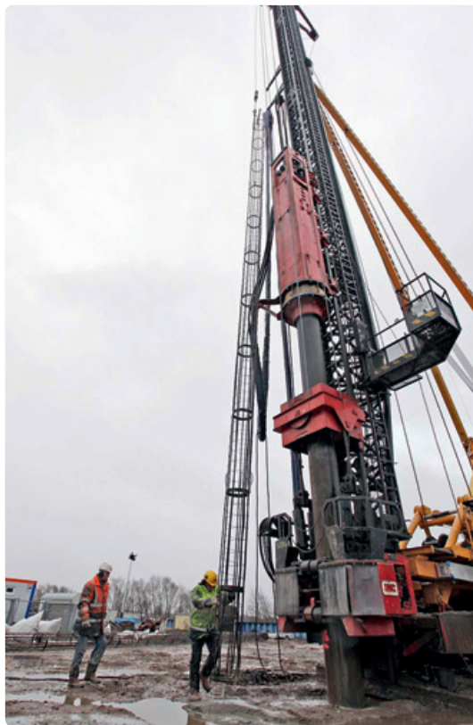
Installing the reinforcing cages
