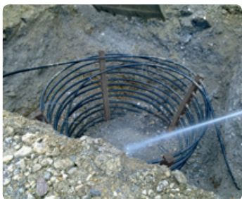
Washing in the filling material
