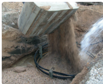
Refilling of the Uponor Energy Cage PE-Xa
