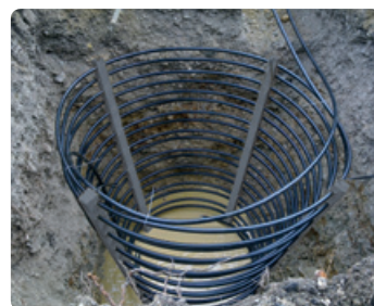
Positioning the energy cage
