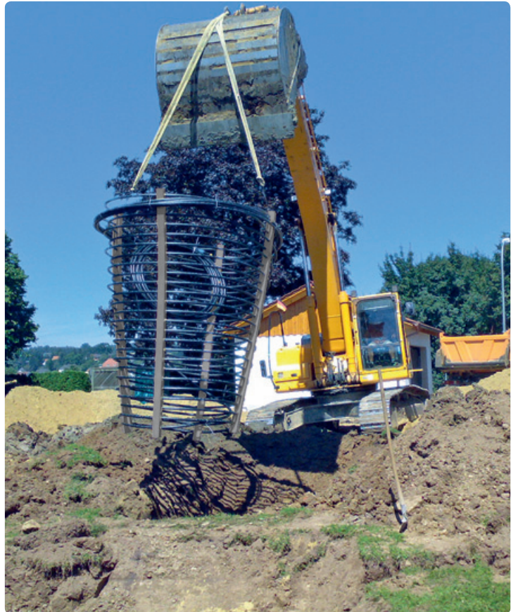
Installation of the energy cage
