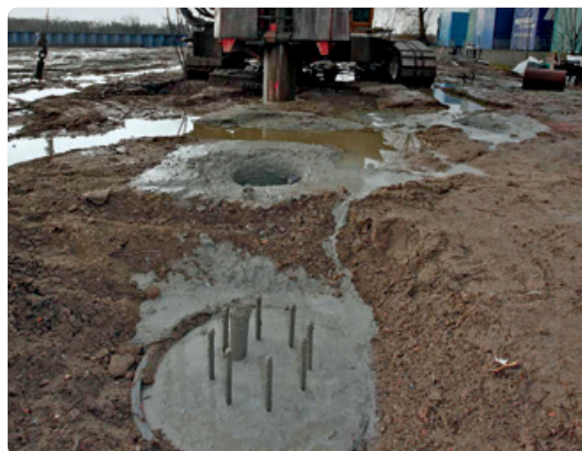
Prefabricated concrete bored pile
