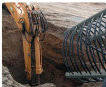
Excavation of the installation pit
