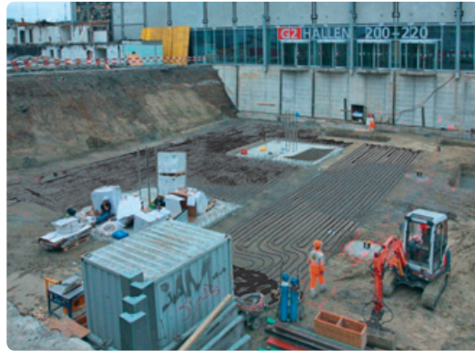
Generation of a floor slab collector
