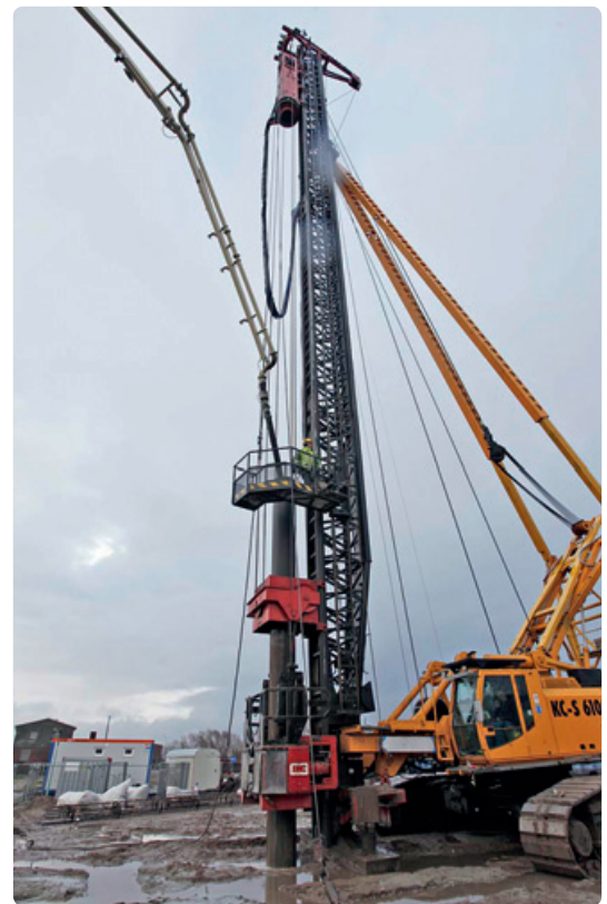
Concreting procedure of the in-situ piles
