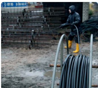
Inserting the PE-Xa pipe loops
