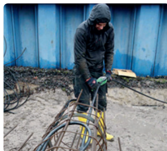
Cutting the inserted pipe loops to length
