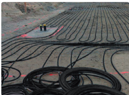
Laying of the individual pipe loops
