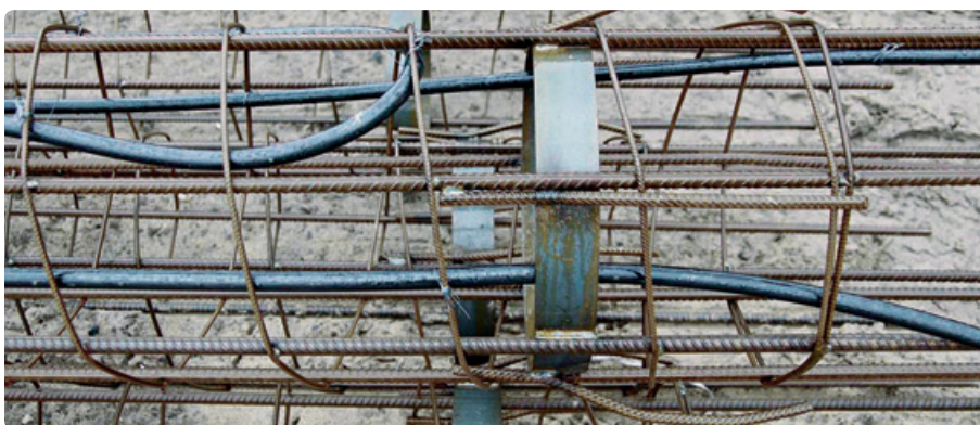
Storage of fitted reinforced cages
