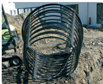
Positioning the connection lines
