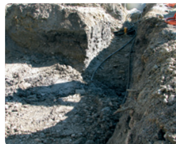
Installed and compacted energy cage
