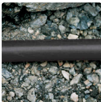
Laying of PE-Xa pipes without sand bed
