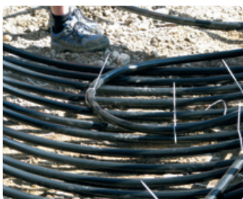
Fixing the flow line
