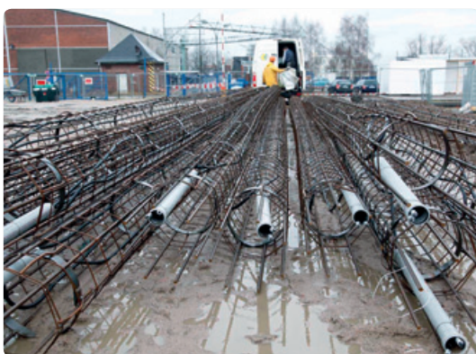
Storage of fitted reinforced cages
