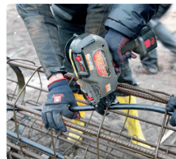
Fixing the pipe loops
