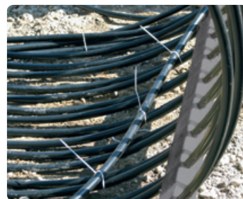
Fixing the return flow line
