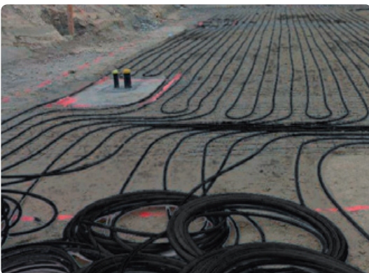
Laying of the individual pipe loops
